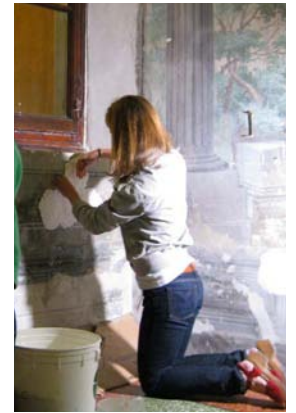
Sophie Scully polycing paint off the wall of the Saletta delle Rovine
