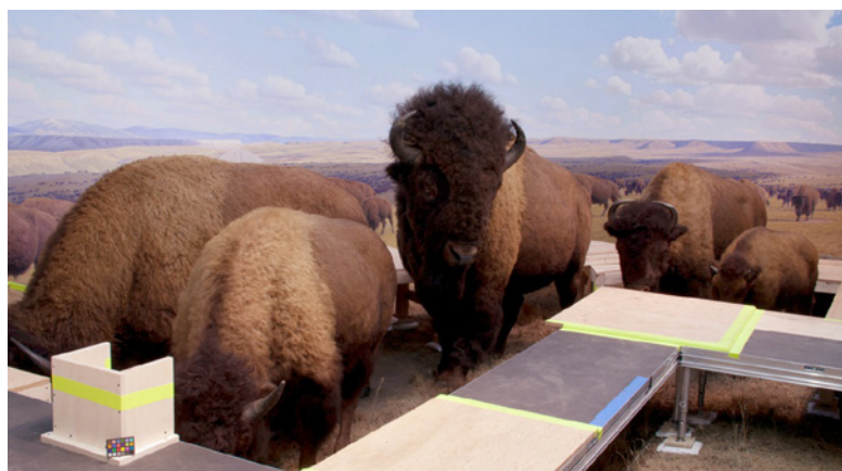
Figure 1. Platforms installed in the bison diorama provide access to taxidermy mounts while protecting fragile foreground elements on the floor of the diorama
